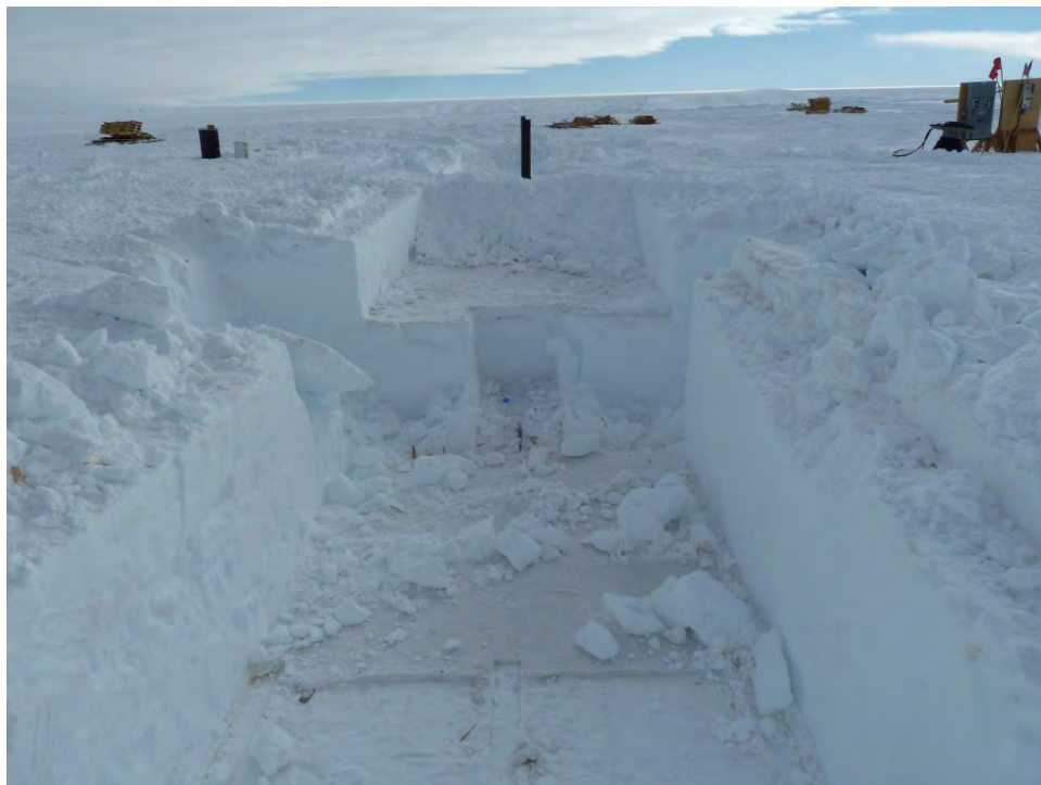
The ice core storage trench after the walls and roof has been removed. The extended borehole casing is in the center upper part of the picture.
